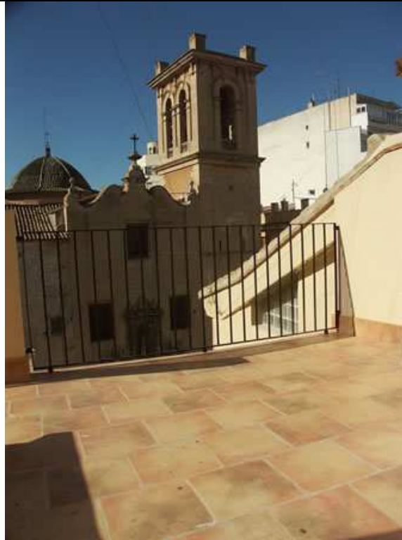
Communal roof terrace
