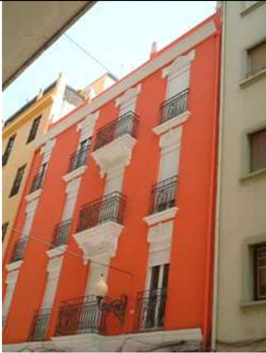
Building – upper levels
